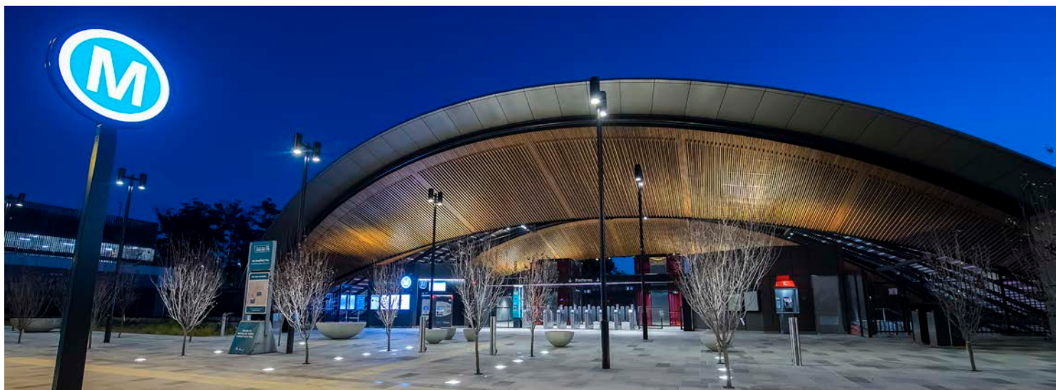
CHERRYBROOK METRO STATION Photo credit: Sydney Metro
